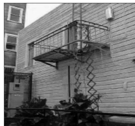
Figure 8. After correction of peeling paint
